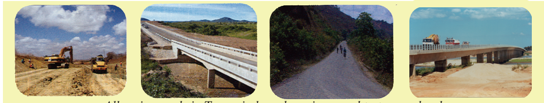
All major roads in Tanzania have been improved to tarmac level
